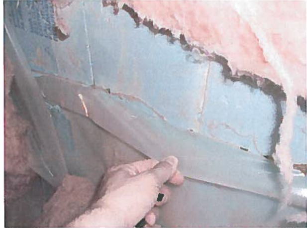
Figure 34: Poly ground cover sealed to wall insulation
