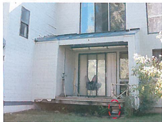
Figure 16: SW porch with added "support"
