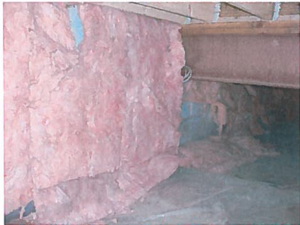
Figure 32: Foundation wall insulation
