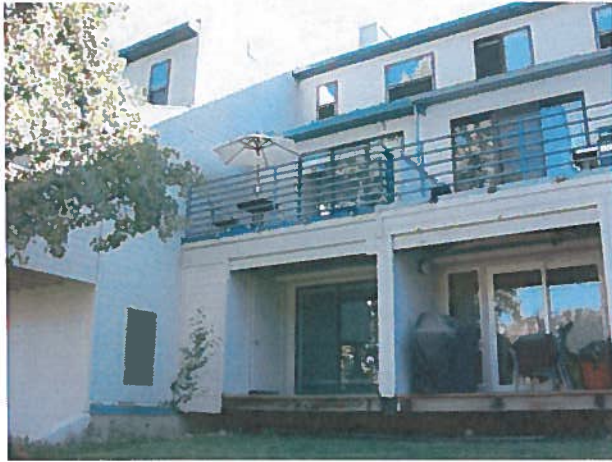
Figure 17: Example of deck over storage closet
