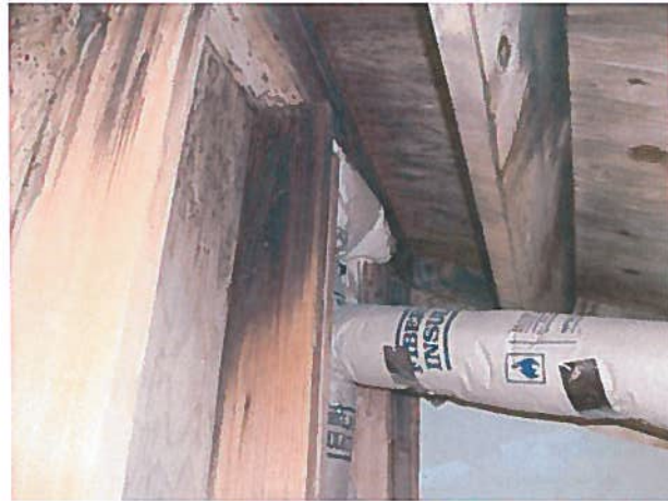
Figure 8: Attic condensation stains at dryer vent
