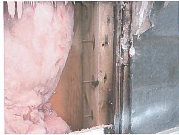
Figure 20: Wing wall attachment to building
