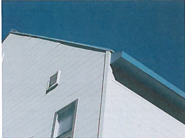
Figure 35: Rake edge at end wall and eave overhang extension
