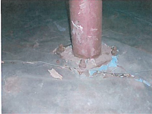
Figure 33: Poly ground cover at lally column
