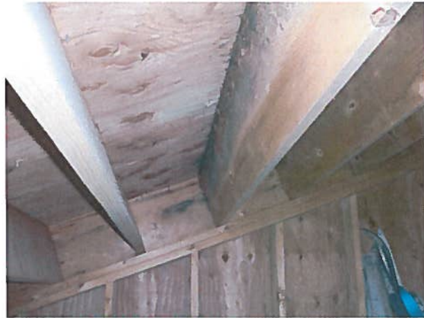
Figure 7: Attic condensation stains
