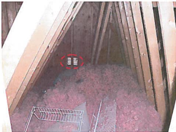
Figure 6: Attic Vent from Interior
