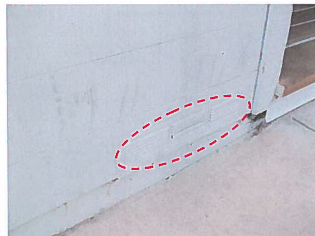
Figure 28: Exterior Basement Vents
